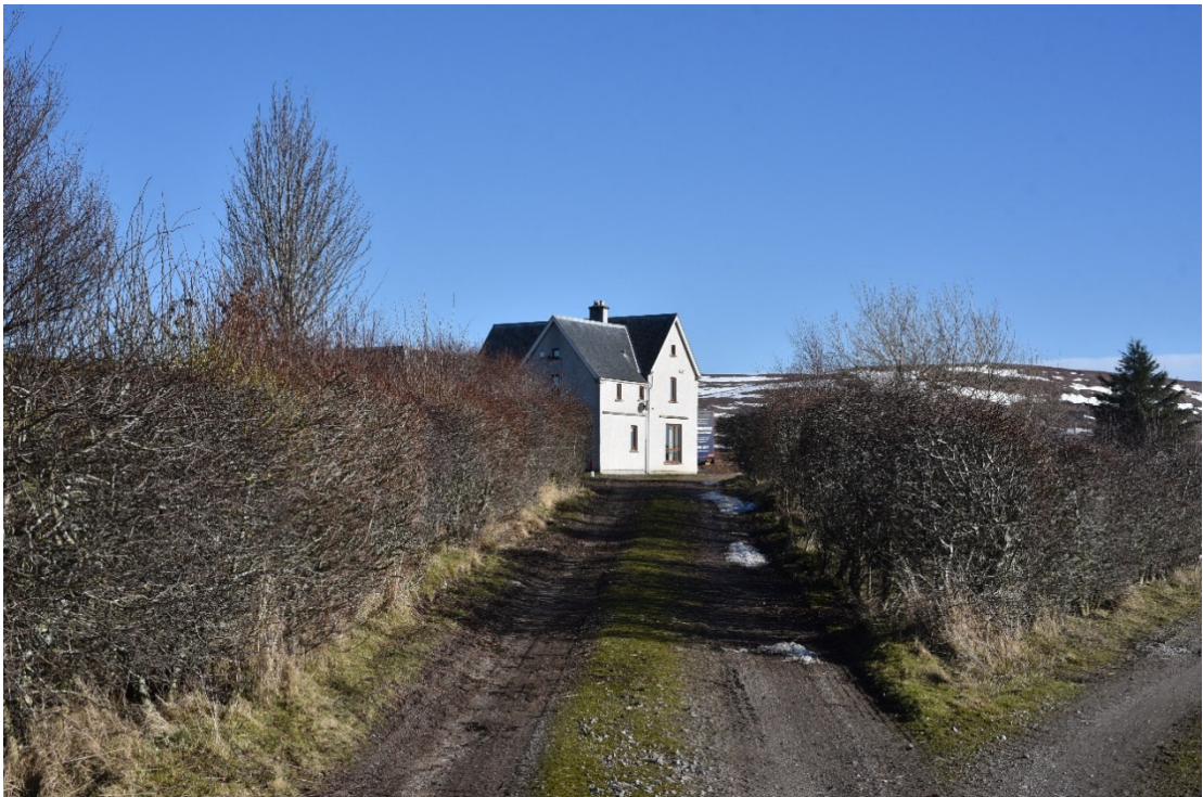
Plate 2 – view north-east from access track towards Dalnessie Lodge (southern façade)
